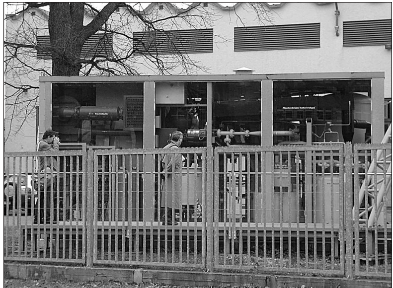
A German Fuel Cell Park features a 250kW natural gas based fuel cell.
